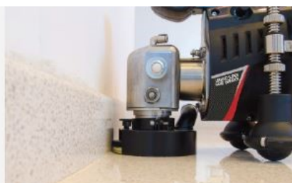
Grinding and polishing perimeters and edges.
