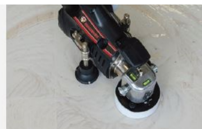
Wet and Dry grinding operation.
