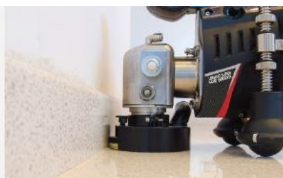
Grinding and polishing perimeters and edges.
